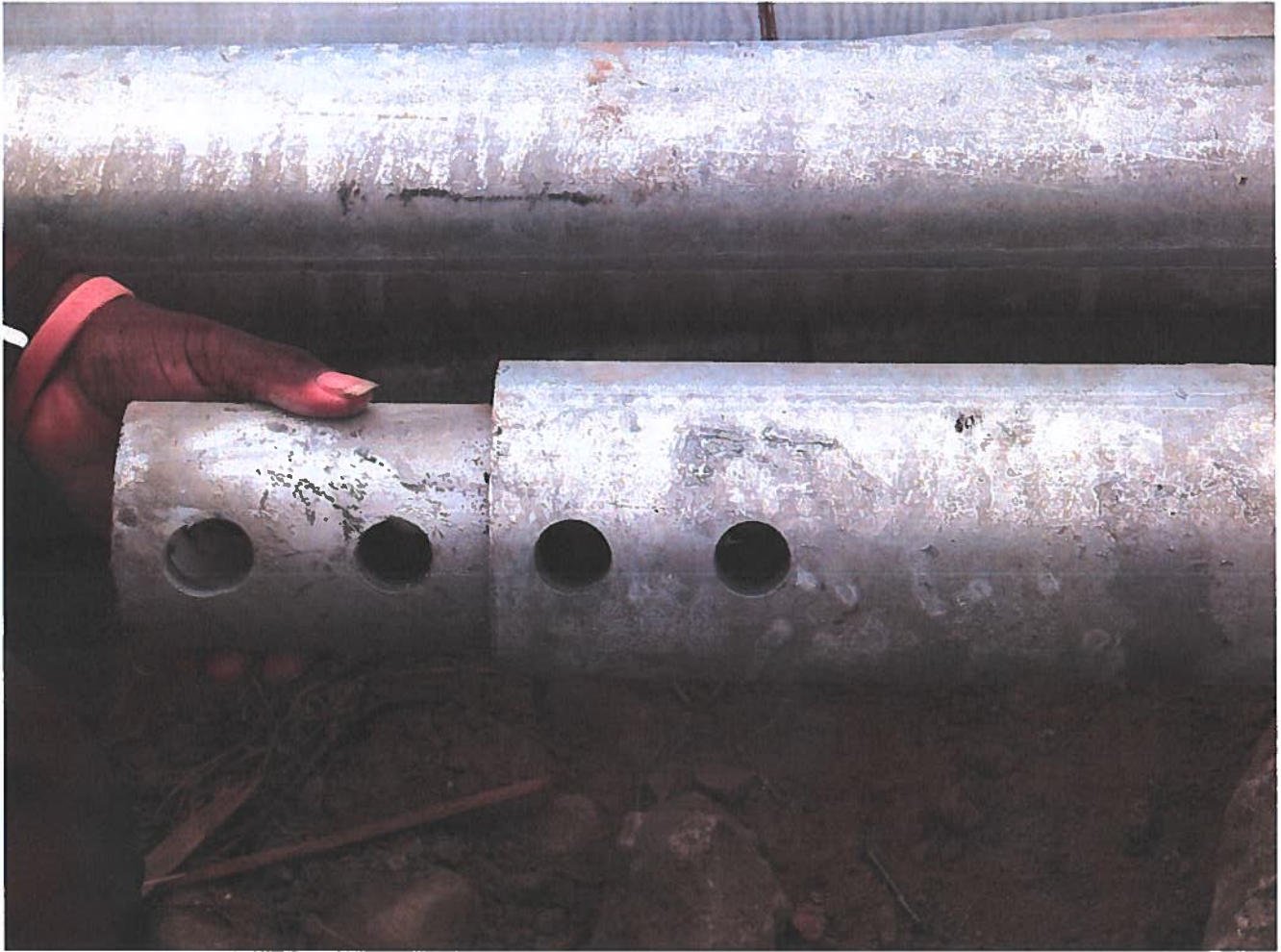
FIG. A-6 Coupling Tube Connected to One Shaft
