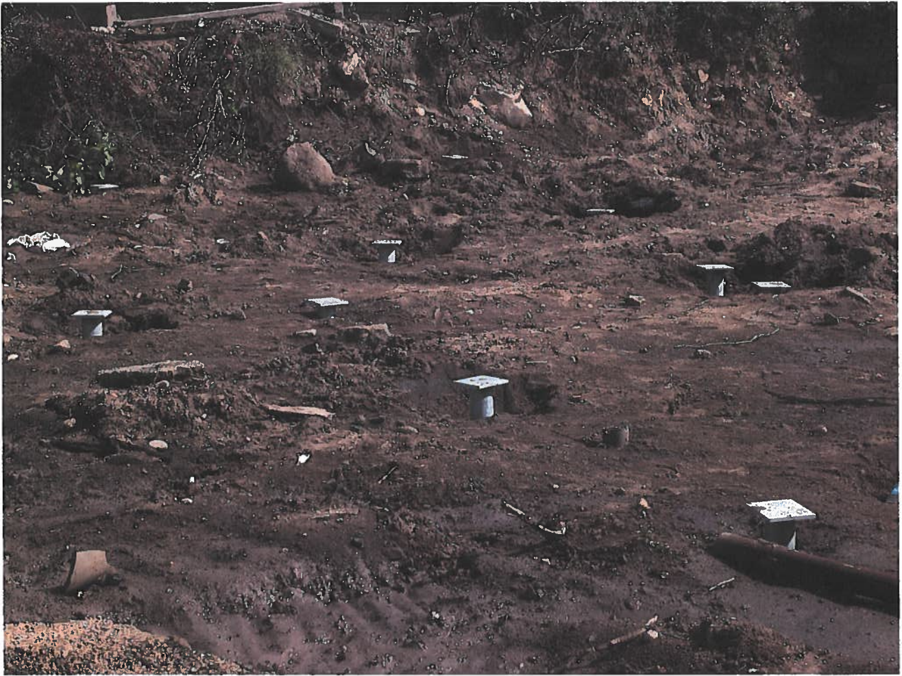
FIG. B-13 Installed Piles with Steel Caps
