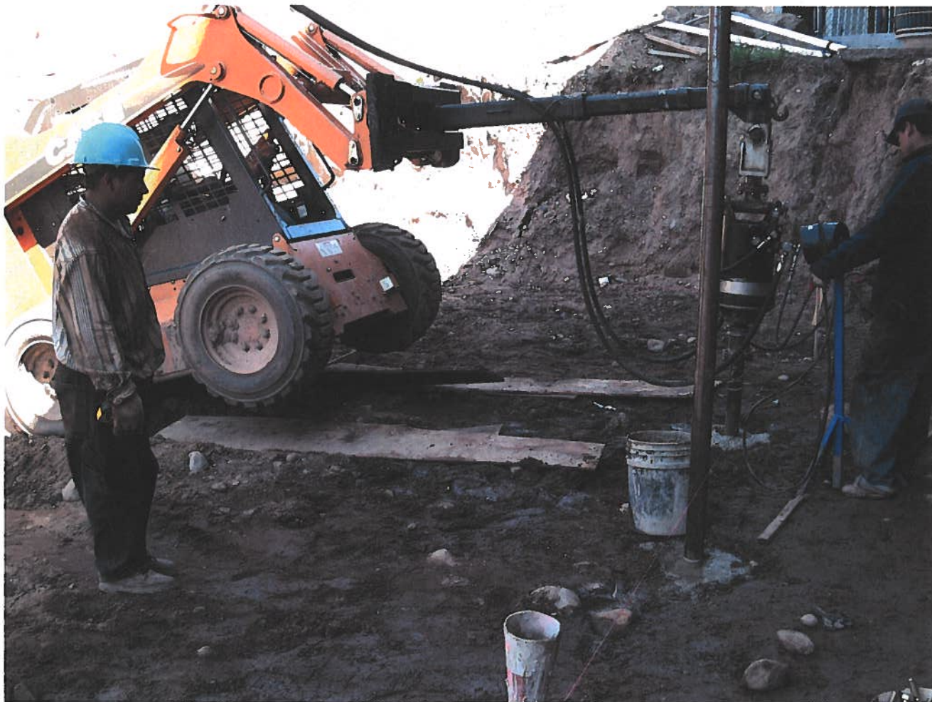
FIG. B-23 Grouted Pile Driving Hole.
