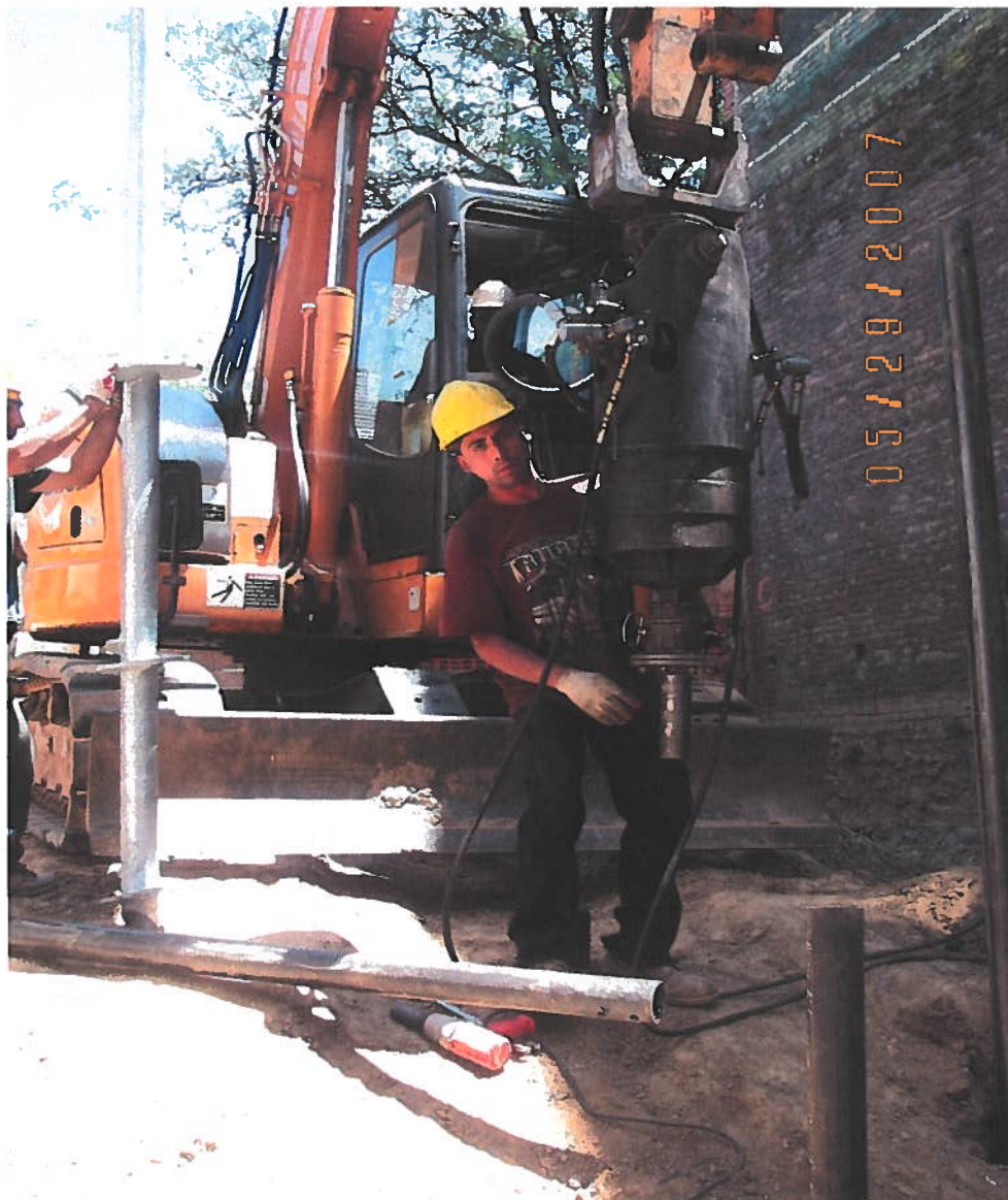
FIG. B-15 Aligning Drivehead
