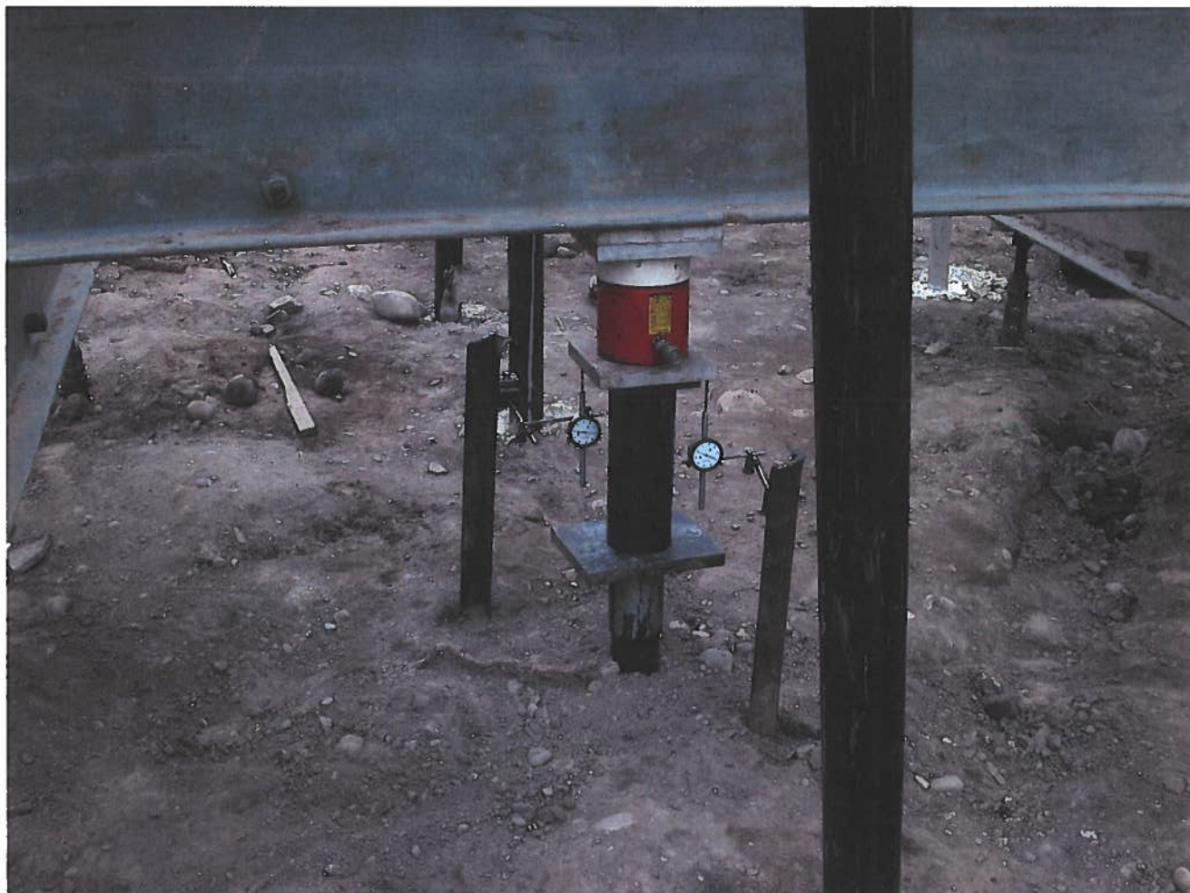
FIG. C-6 Pile Load Test Loading Frame over Test Pile
