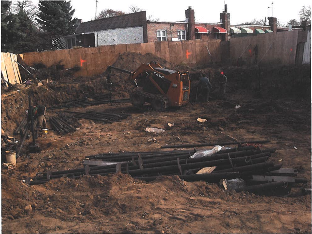
FIG. B-5 Pile Installation Driving Pile.
