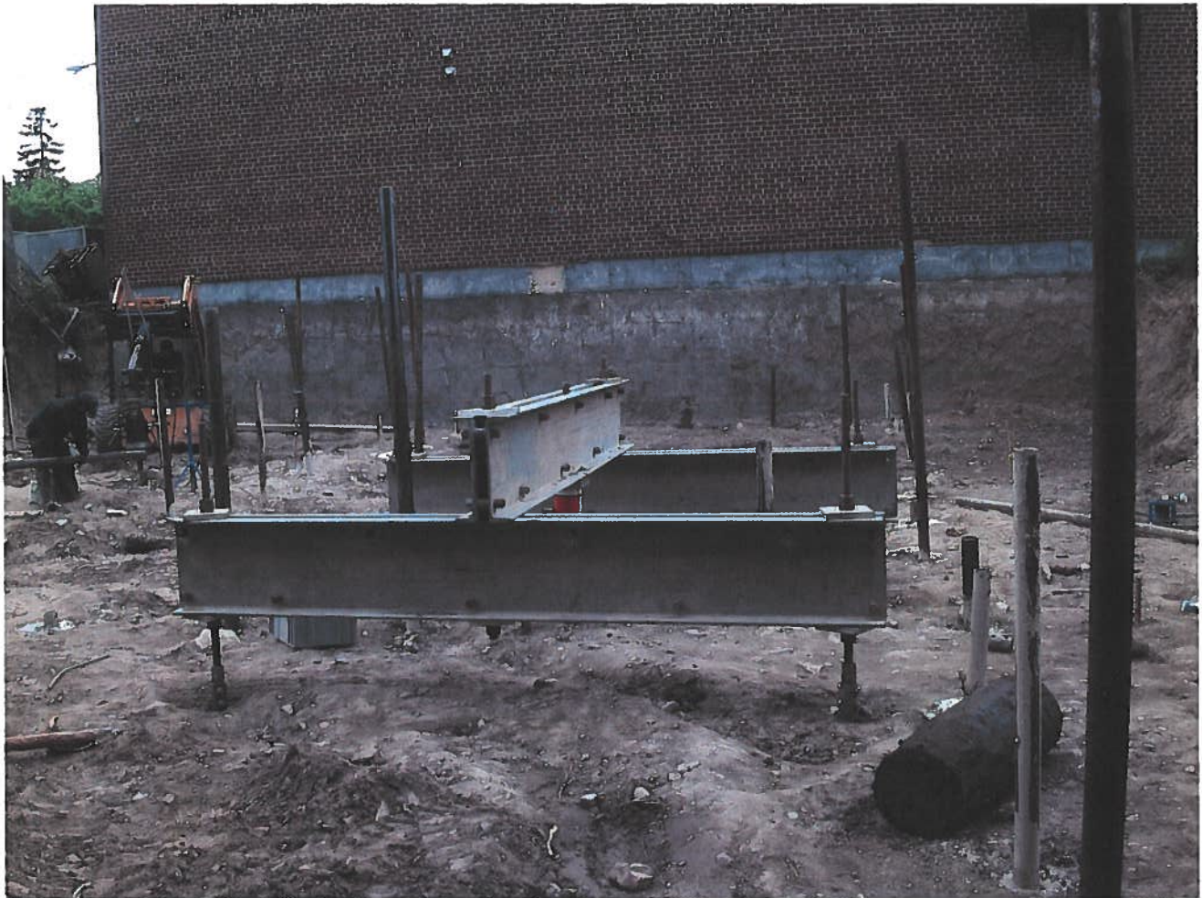
FIG. C-2 Pile Load Test Framing Beams
