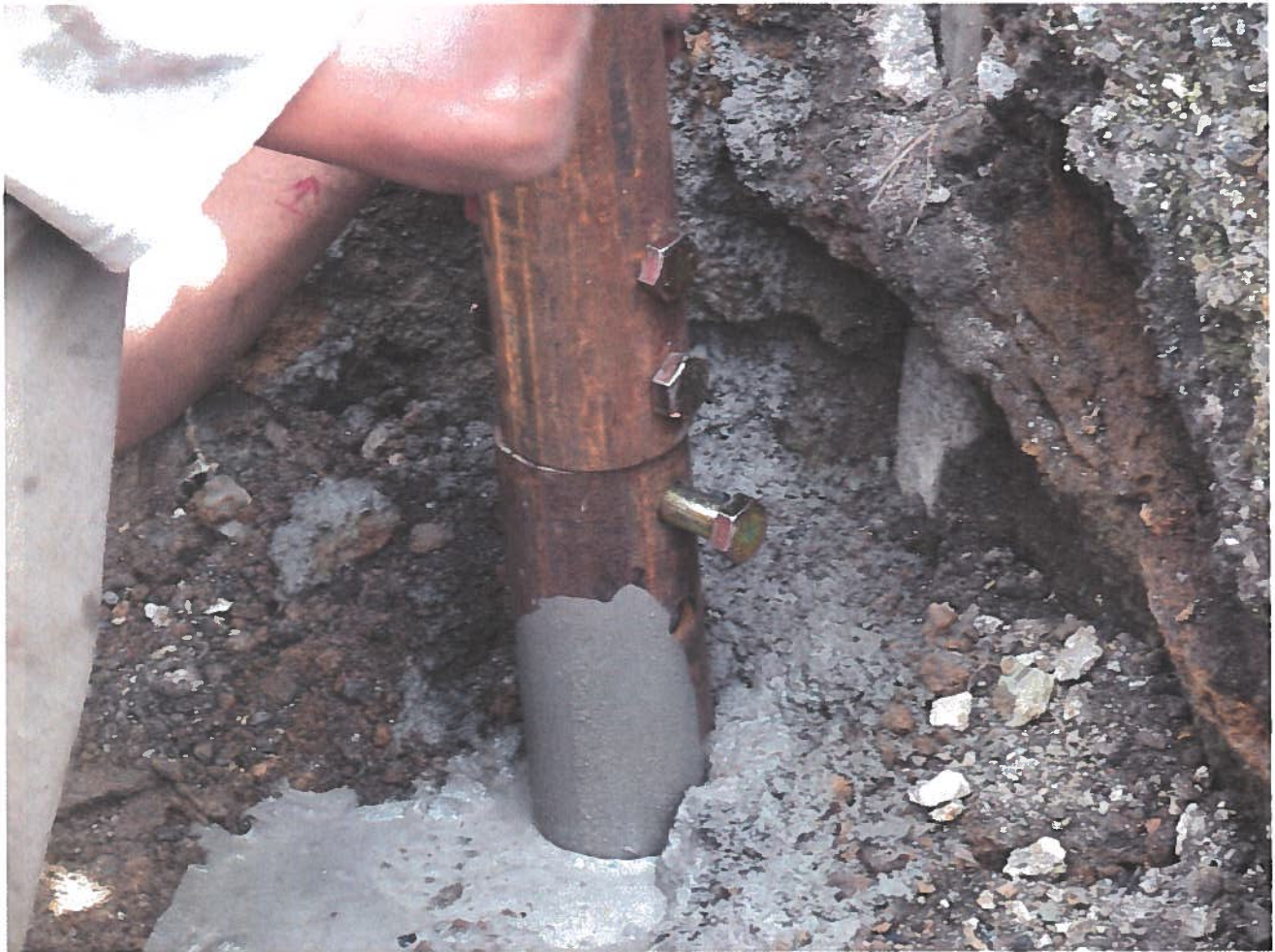
FIG. B-27 Grouting Hole around Pile during Installation.
