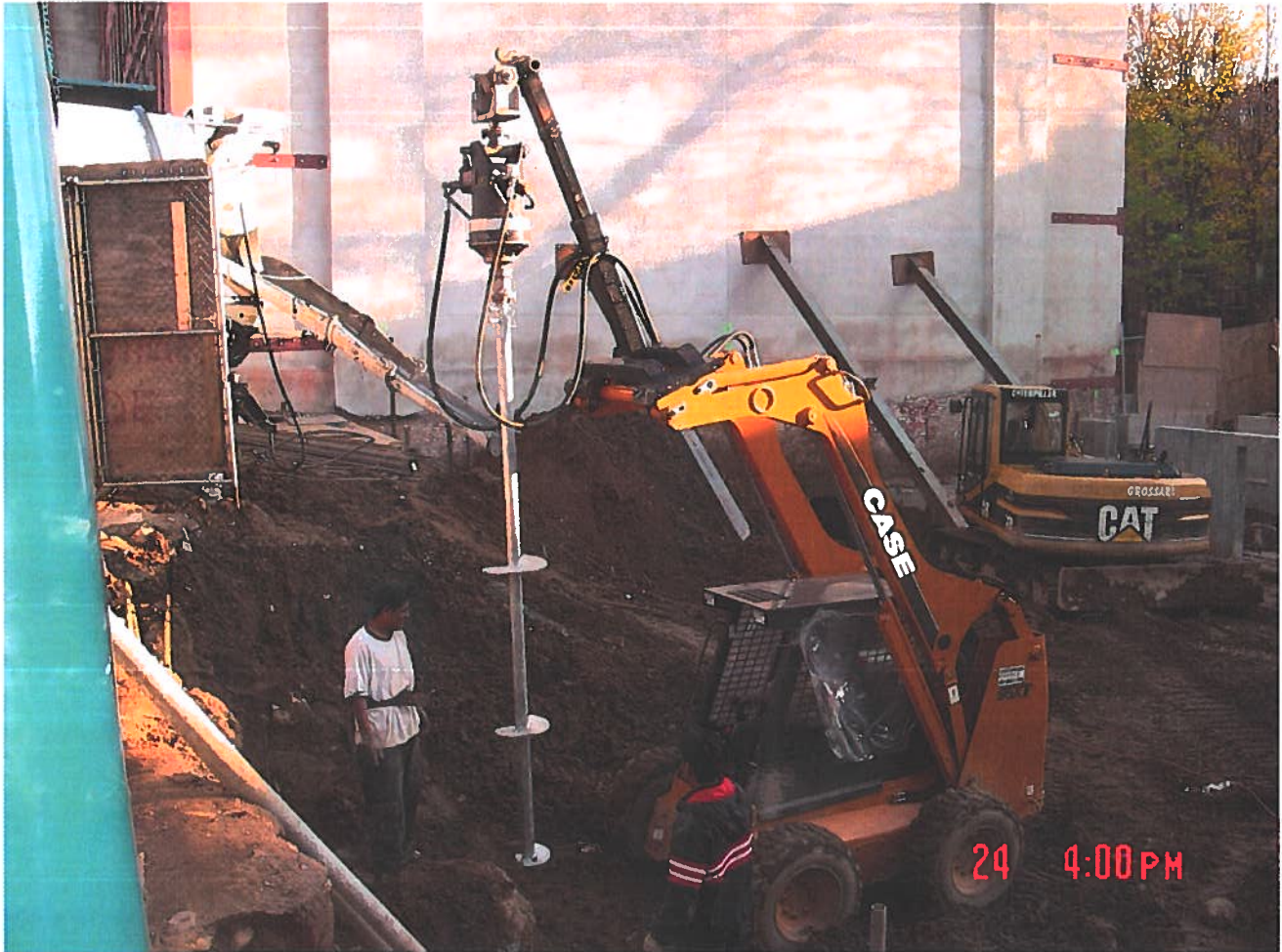
FIG. B-34 Vibration-free Helical Pile next to Shored Building.
