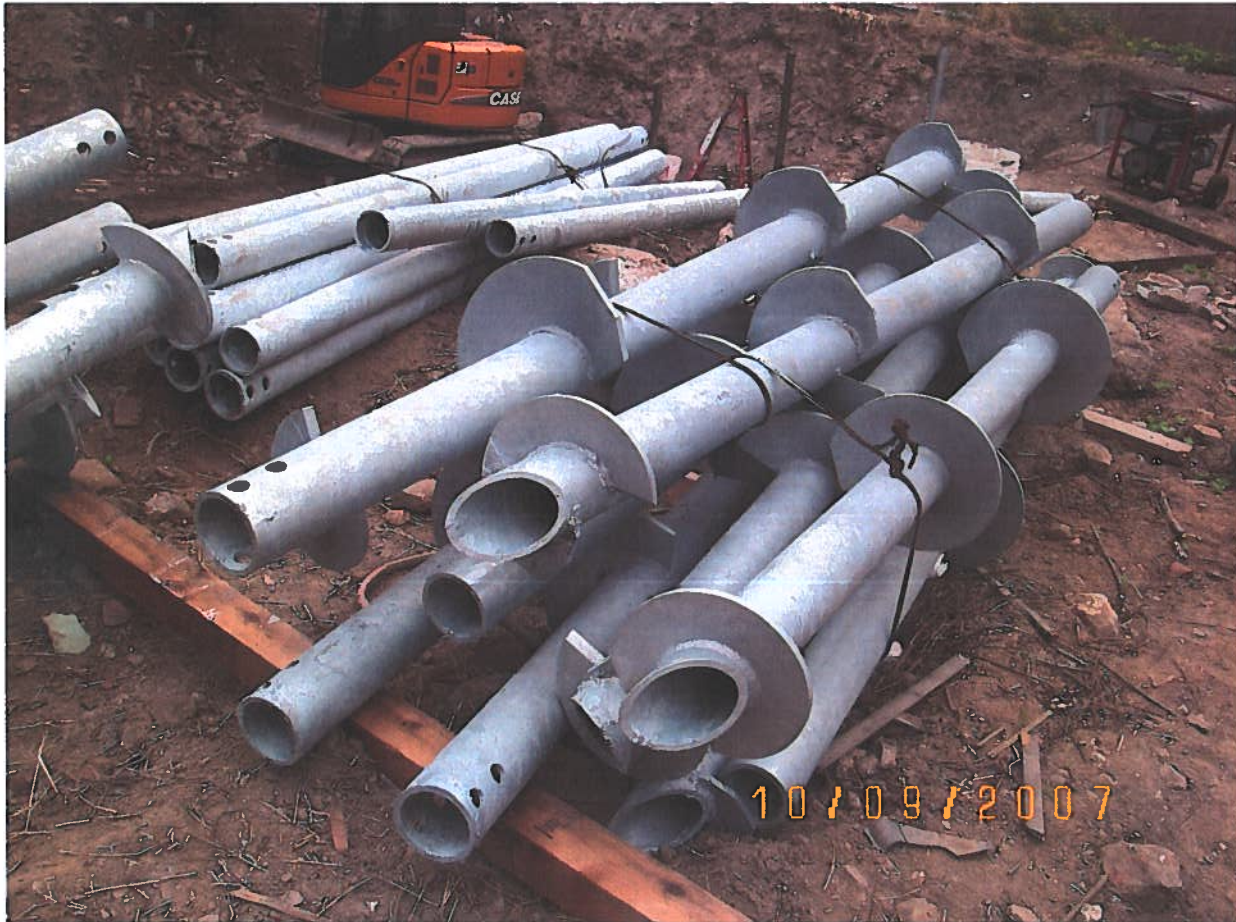
FIG. A-2 Piles at The Job Site
