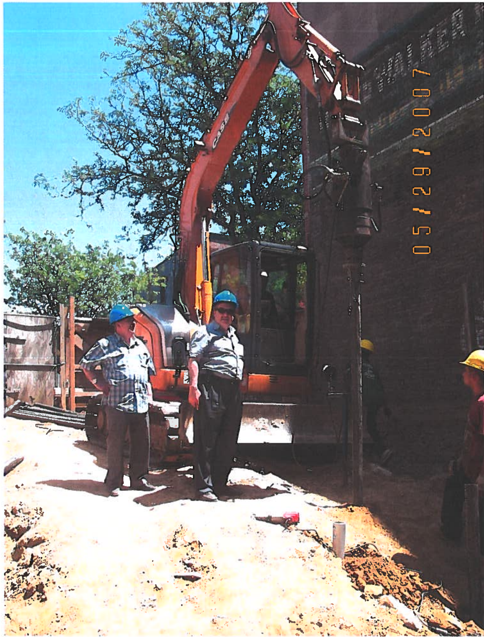
FIG. B-14 Engineers Inspecting Pile Installation
