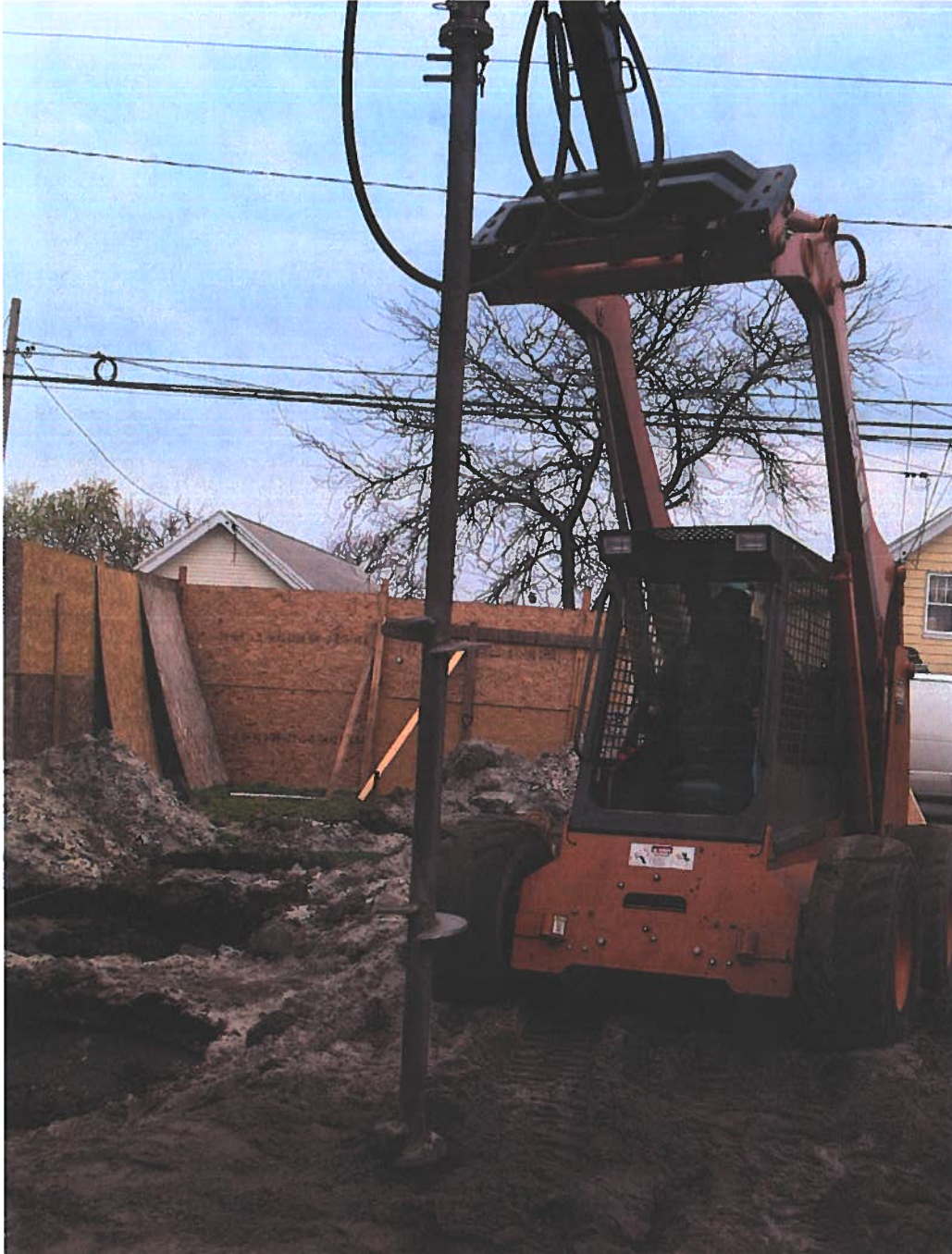
FIG. B-8 Pile Installation Project 3
