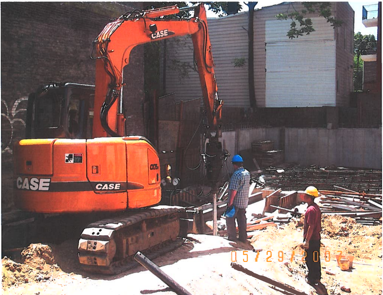
FIG. B-16 Driving Piles Around Shoring
