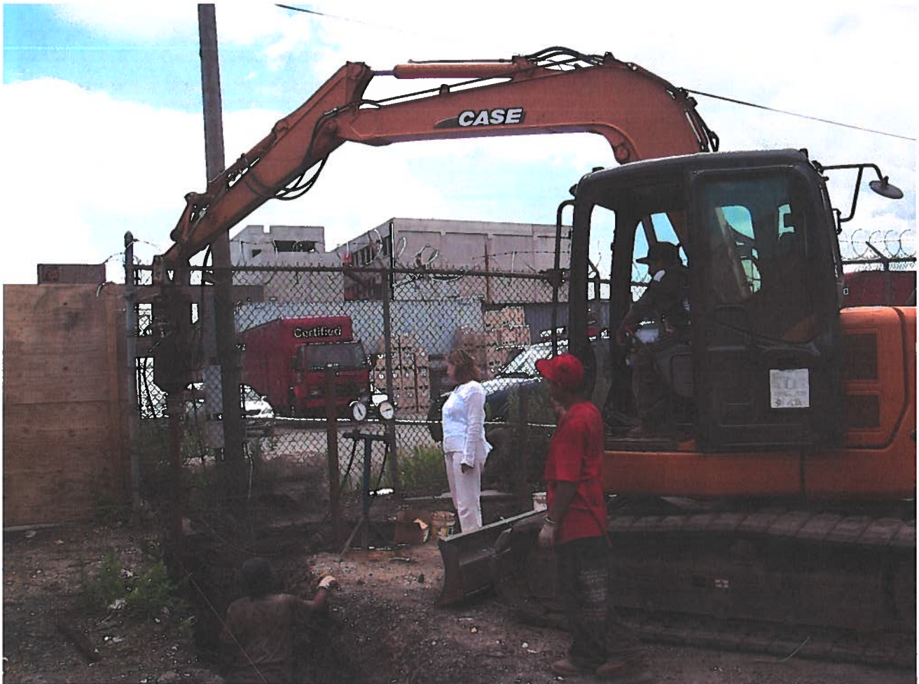
FIG. B-30 Pile Installation and Monitoring Operation.
