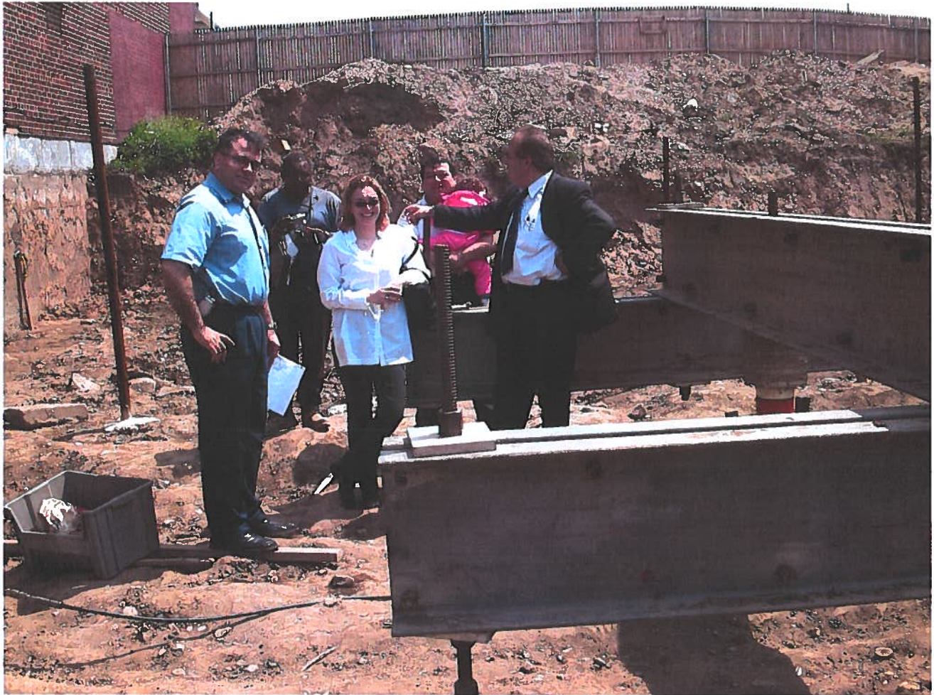
FIG. C-1 Pile Load Test Set Up
