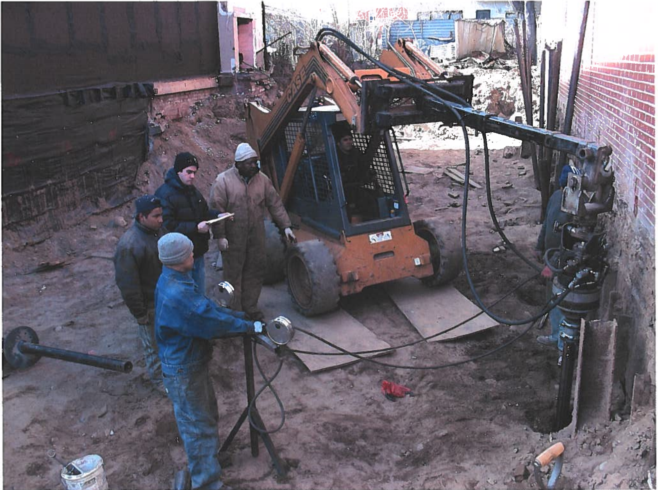
FIG. B-11 Pile Installation Last Extension
