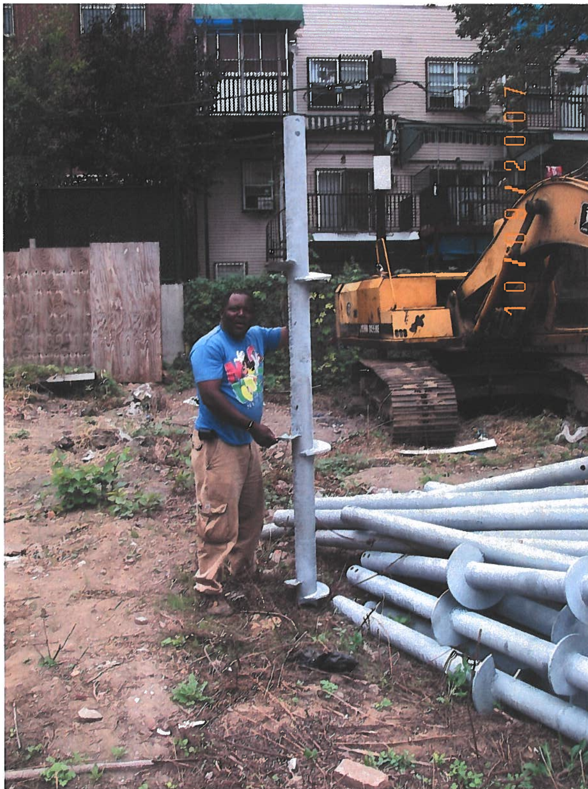
FIG. A-1 Starter Section with Three Helices
