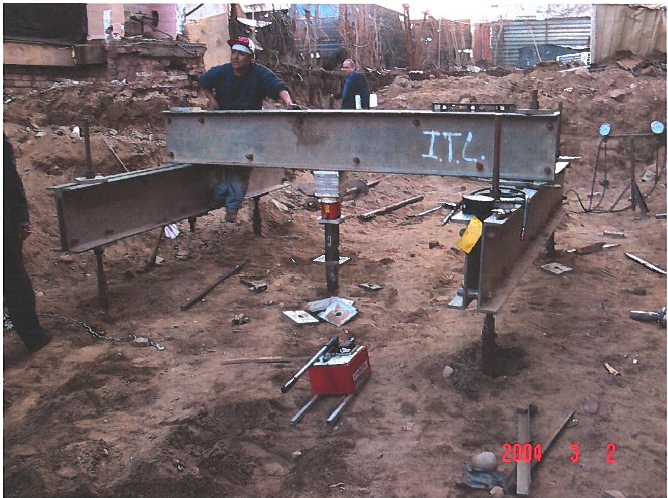
FIG. C-3 Pile Load Test Framing Beams Held by Four Anchor Piles
