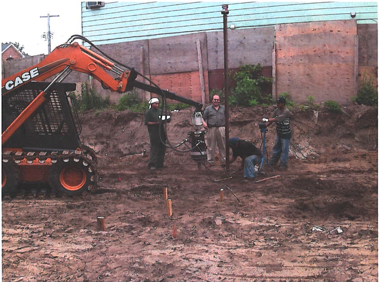
FIG. B-10 Pile Installation Connecting Two Sections
