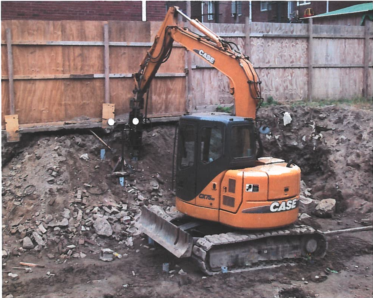
FIG. B-43 Pile Installation Equipment
