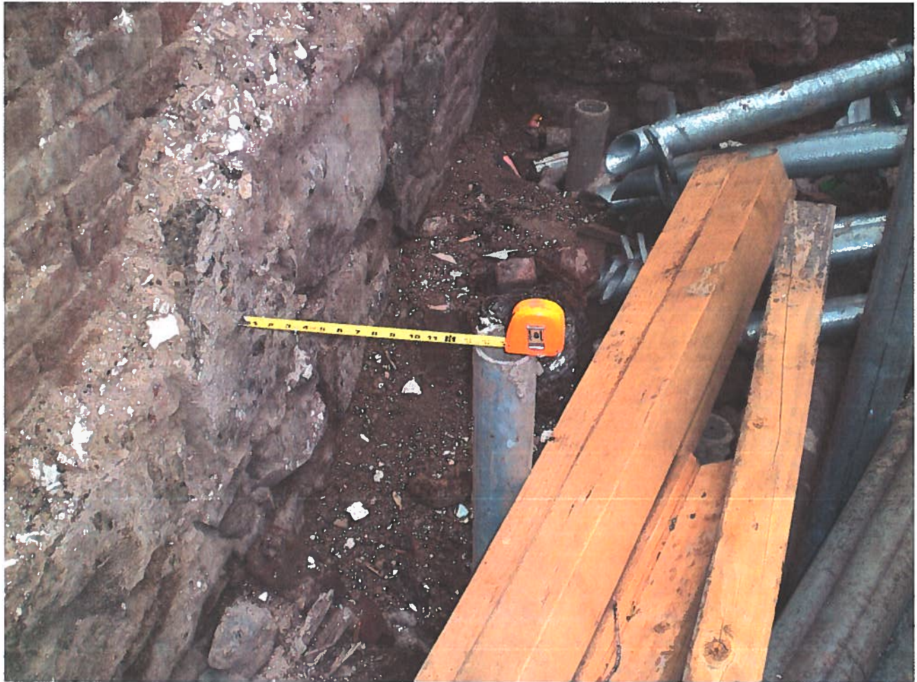
FIG. B-36 Clearance for drivehead.(12"-18")
