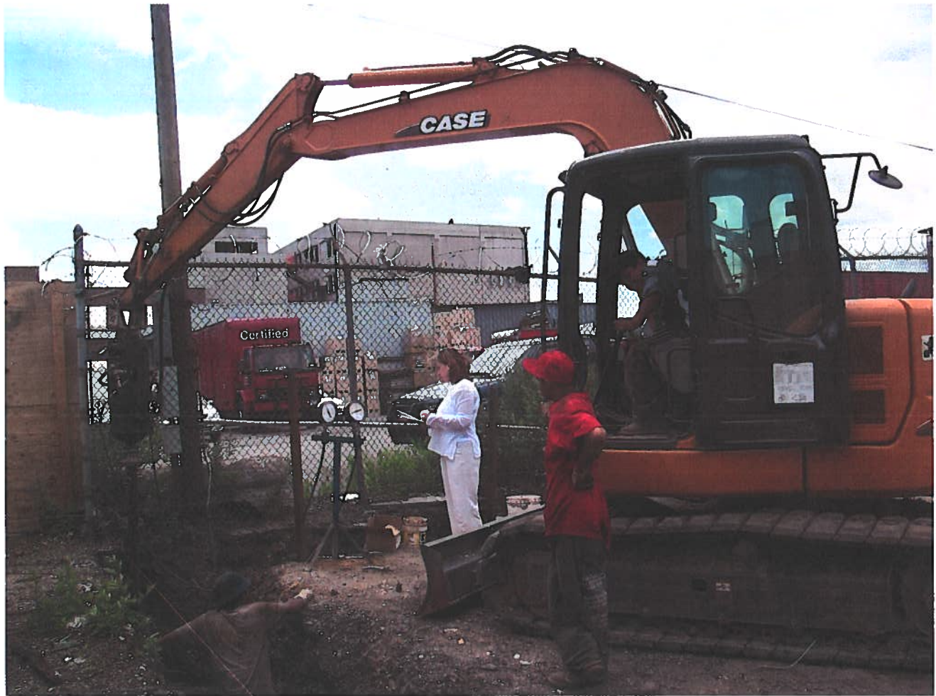
FIG. B-6 Pile Installation Project 1
