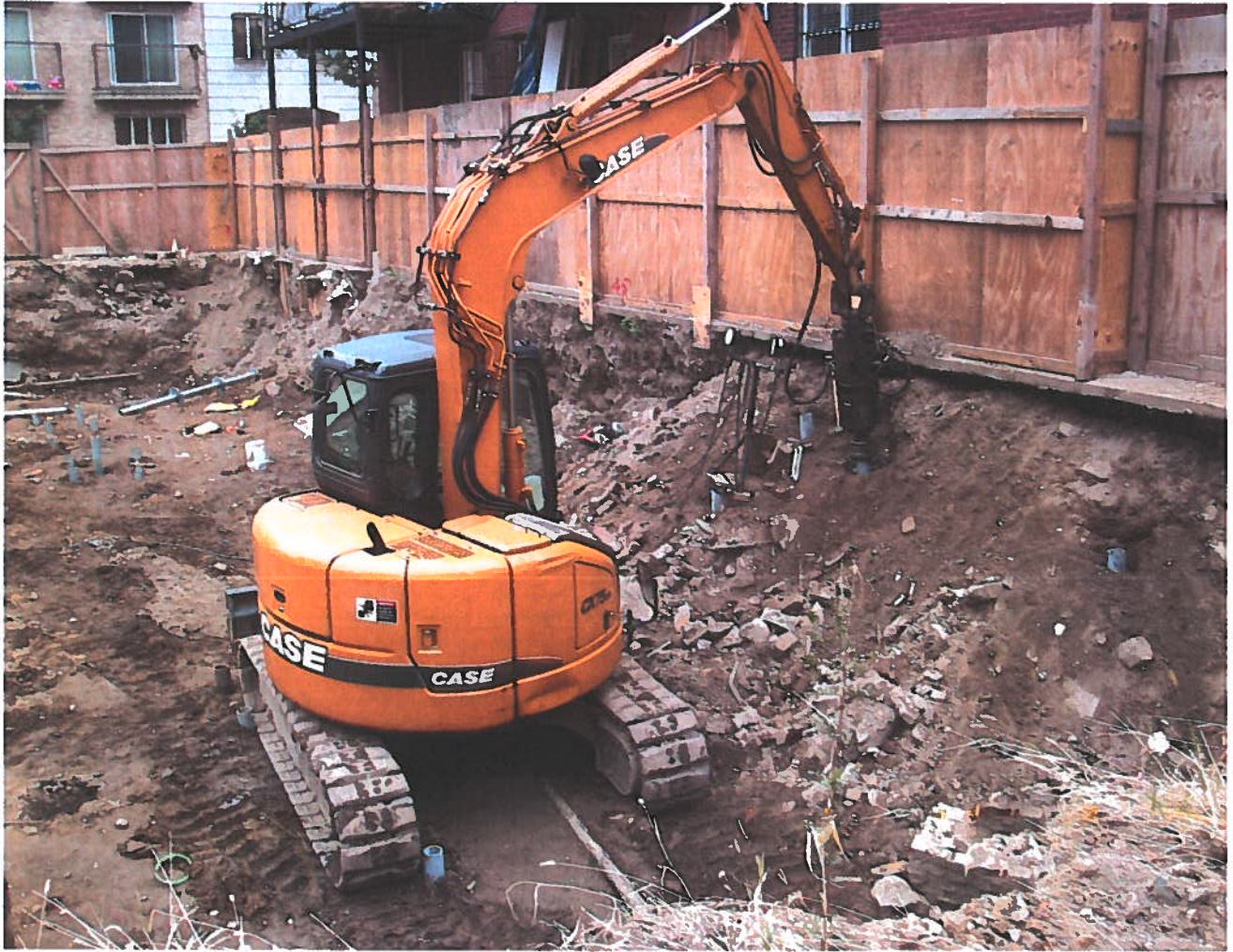
FIG. B-44 Pile Installation Equipment
