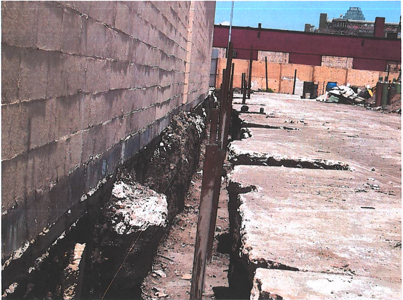
FIG. B-22 Excavated Trench to be Used for Pouring Concrete Pile Cap. Piles to be Cut-off.
