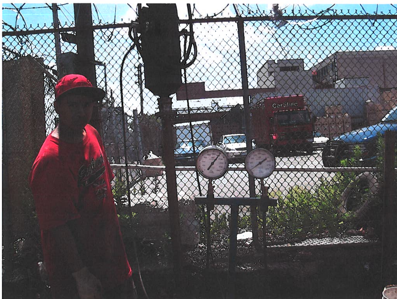
FIG. B-28 Pile Installation Pressure Monitoring.
