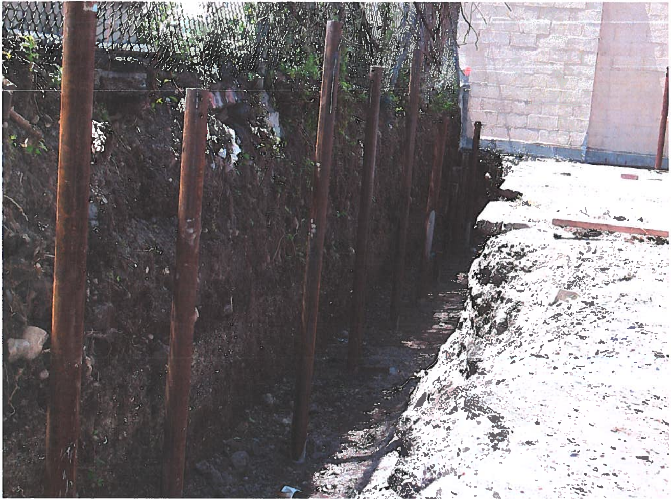
FIG. B-20 Piles in Line for Wall Foundation
