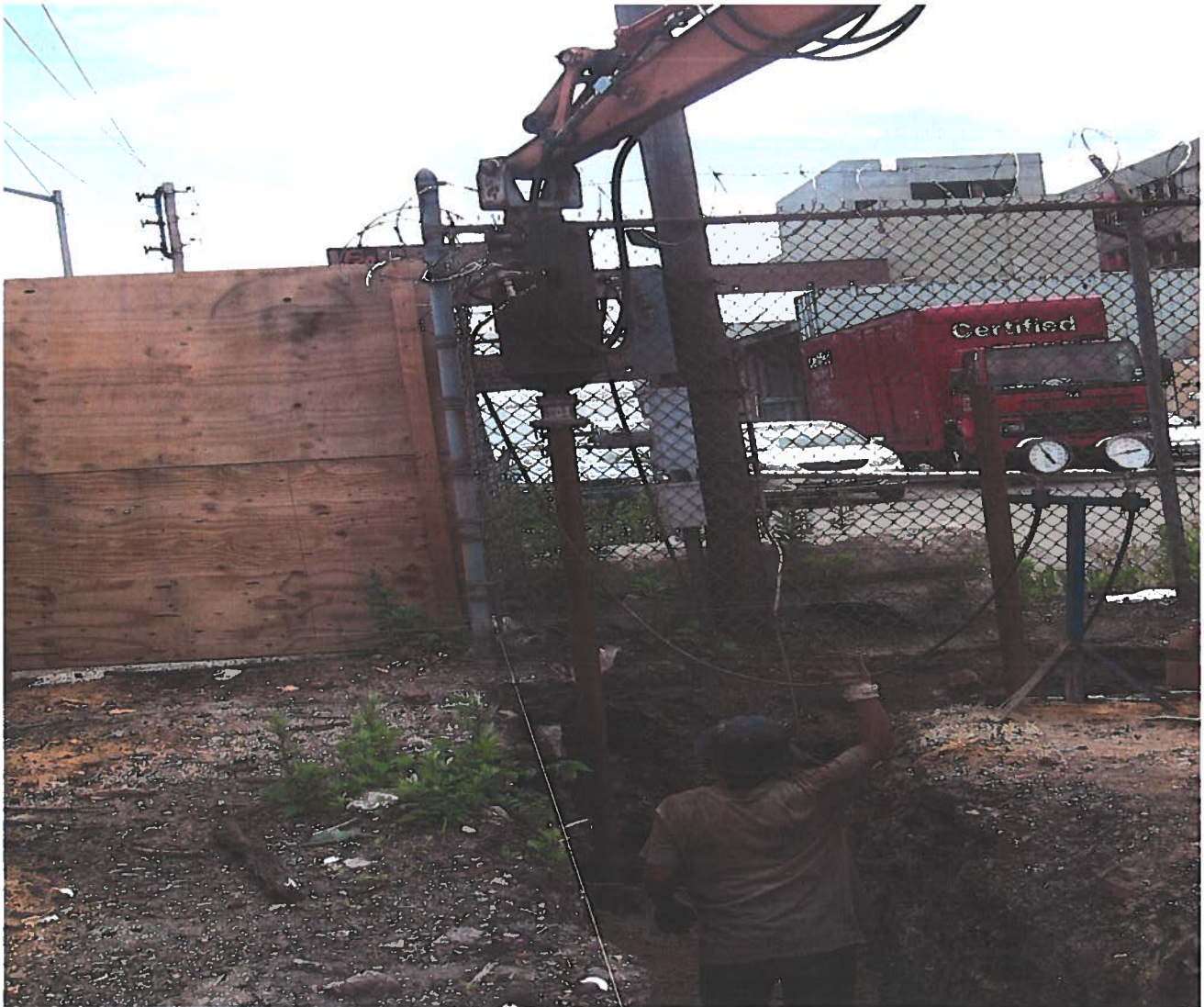
FIG. B-32 Aligning Corner Pile.
