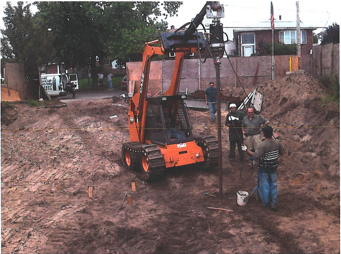
FIG. B-24 Hooking up Lines for Measuring Pressure during Pile Installation.
