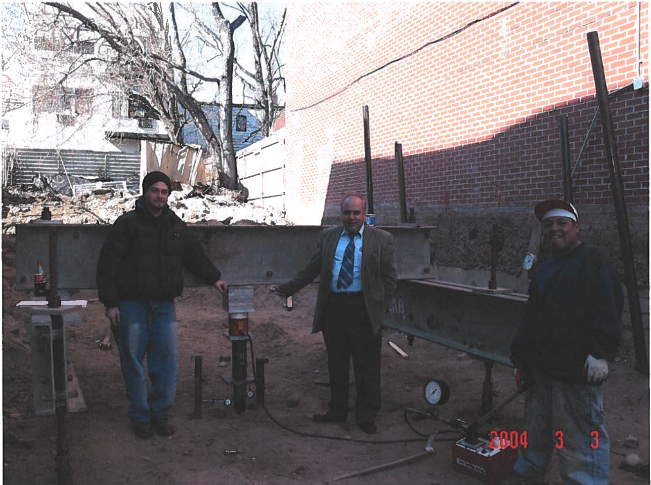
FIG. C-4 Pile Load Test Load Frame Test Pile and Hydraulic Jack
